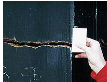
Signs of panel zone deformation
